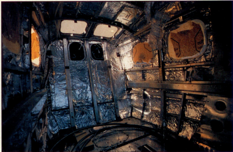
P210 cabin is laid bare, and foil-backed foam soundproofing is glued to metal surfaces.
